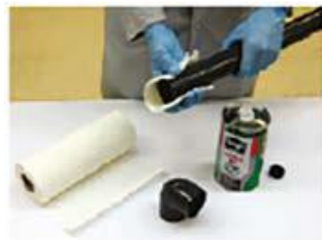
Cleaning the pipe and the socket
