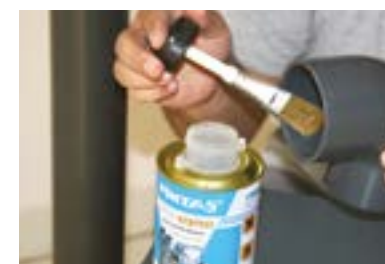
Applying the adhesive
