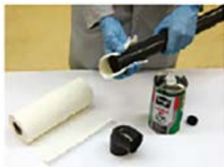
Cleaning the pipe and the socket
